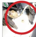
Locate the brass nut connecting the fluid pipe to the heat exchanger. Then loosen with a spanner so that the pipe can be removed as shown.
